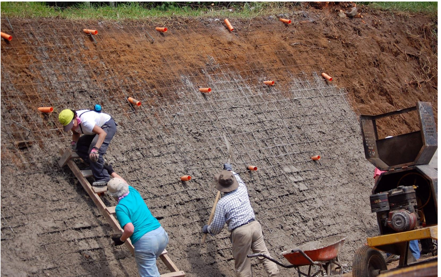
Cementing the retaining wall
