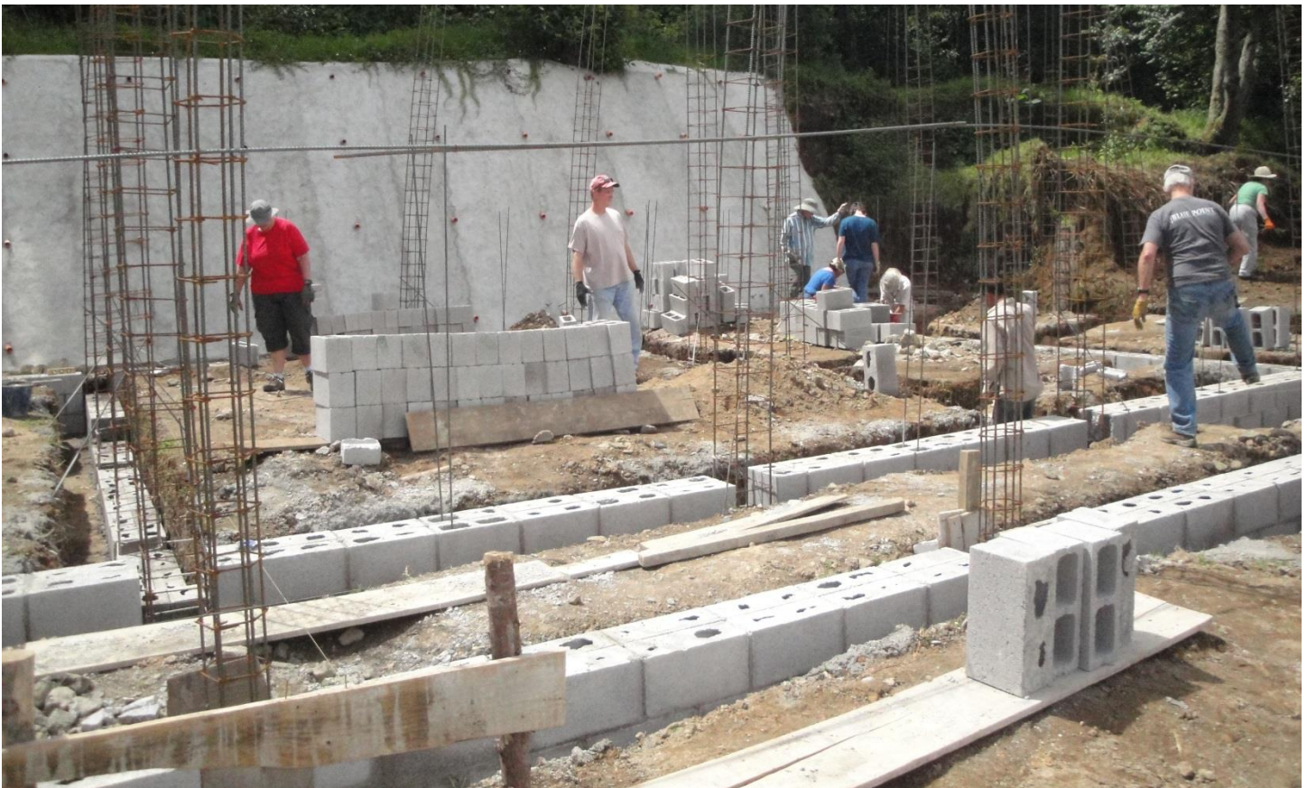
Completing the foundation
